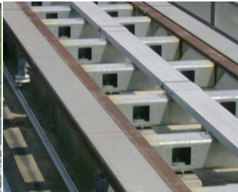
Fig. 2 Typical arrangement for LIM Gw regardless if it is used either rubber tired, steel wheeled or levitated vehicle
