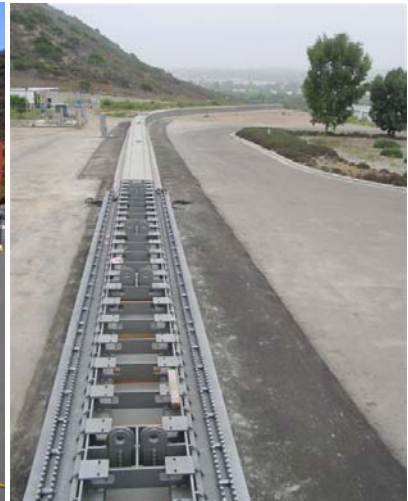
Fig. 12 LSM Guideway @ San Diego
